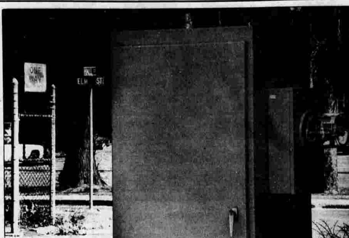
RESTORATION SNAG — A planned wall enclosure for this light-control box off Hall Court has contributed to a snag in restoration plans for historic Cheney Hall.
